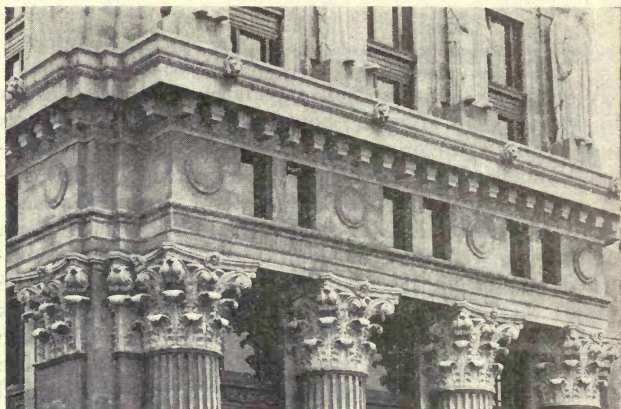
FIG. 91—CAPITALS AND CORNICE (WITH LION HEADS) OF CONCRETE STONE, BOSTON CITY HALL ANNEX—EMERSON & NORRIS CO.
